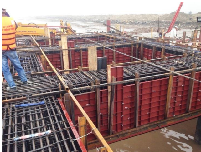
Nam Dinh Vu wharf (Hai Phong)
