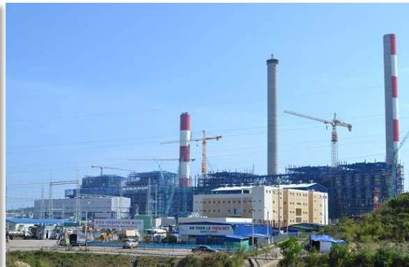
Mong Duong 1 & 2 Thermal Power Plant (Quang Ninh)
