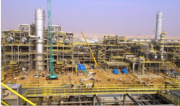
Nghi Son oil refinery (Thanh Hóa)
