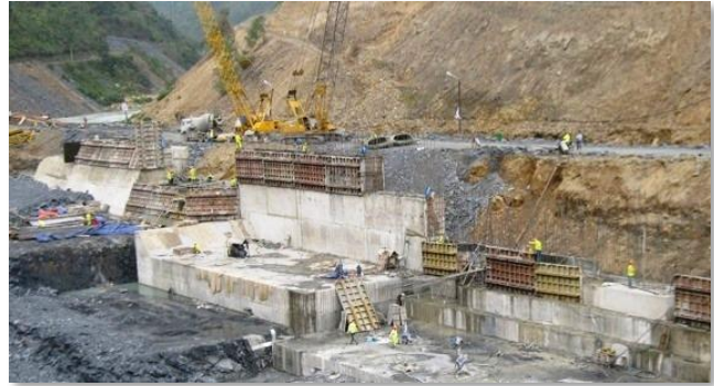
Bac Me hydropower project (Ha Giang)
