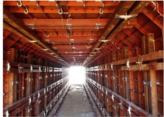
Water treatment factory (Hoa Lac Hi-Tech Park)
