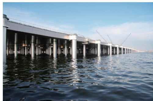
図1 海洋鋼構造物へのSUS鋼被覆の適用 Application of SUS sheathing to offshore steel structures
