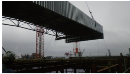
(b) Construction of movable roof
