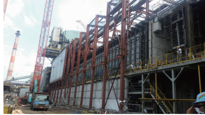
(e) Demolition of temporary building
