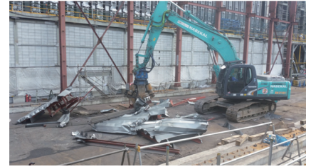
(f) Cutting of movable roof
