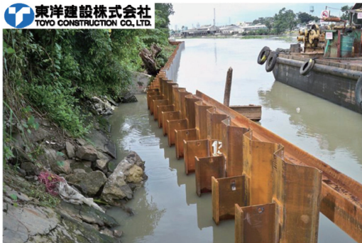
写真5 フィリピン／護岸工事でのハット+H矢板の施工状況 Application to river revetment in Philippines (during construction)
