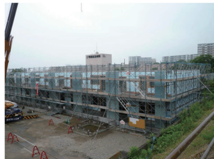
(b) Construction of second-story
