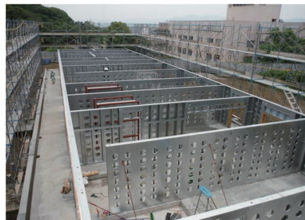
(a) Construction of first-story
