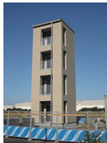
写真11 4階建て試作棟 4-story experimental building
