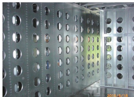
(c) Inside structure
