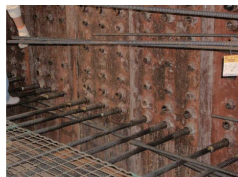
写真4 鉄筋の接続状況 Connection situation of the reinforcing bar
