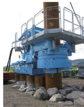
(a) Surging the rubbles by Gyropress method
