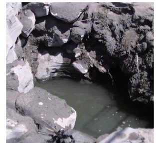
(b) Hollowed rubbles by Gyropress method
