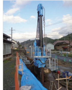
写真 12 道路擁壁適用状況 Condition of application for retaining wall
