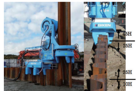
写真6 打設試験結果(圧入工法) Condition of hydraulic jacking driving
