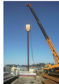
写真 13 仮設土留め適用状況 Condition of application for temporary retaining wall
