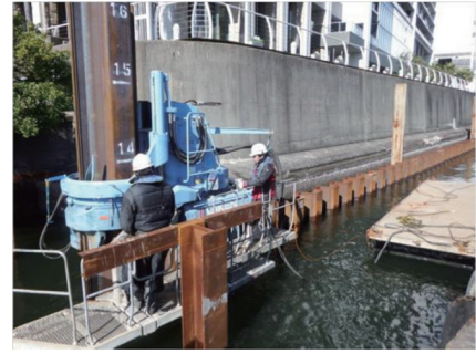
写真 11 河川護岸 (防潮堤) 適用状況 2) Condition of application for river revetment
