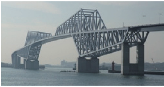
写真5 SBHS を用いた橋梁 Steel bridge built of SBHS
