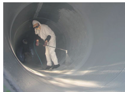
写真8 COG配管内面の防食塗装の施工状況 Internal coating application of developed non-solvent paint to COG pipeline
