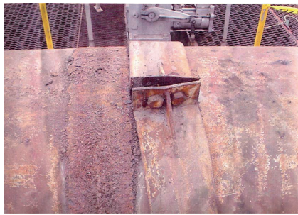
写真9 管台の鋼製バンド下のすきま腐食 Crevice corrosion under pipe supporting bands
