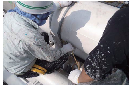
写真10 管台防食の施工状況 Anti-corrosion coating into the gap under pipe supporter and bands
