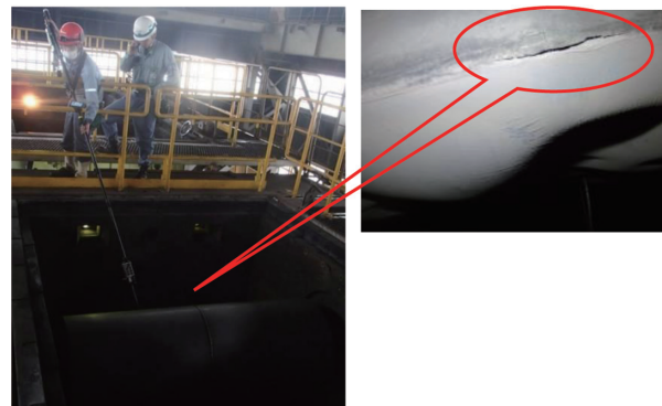
図9 連続焼鈍炉防熱板亀裂点検への適用状況と撮像写真 (2015年4月) Inspection and captured image of insulation plate crack in C.A.P.L. (at 2015.4)
