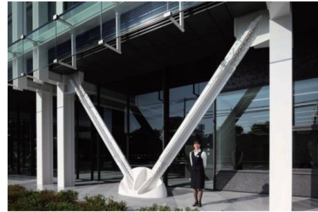
図7 制振ブレースとBT-HT880適用柱 Appearance of energy dissipative brace and column applied BT-HT880
