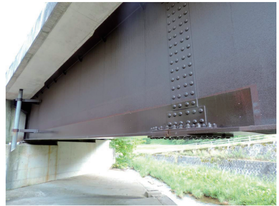
図 17 補修塗装事例 Example for repaired painting
