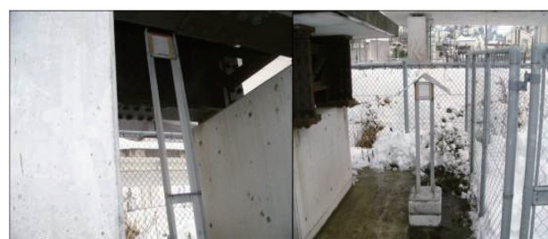
(a) Inside of the bridge (b) Outside of the bridge
