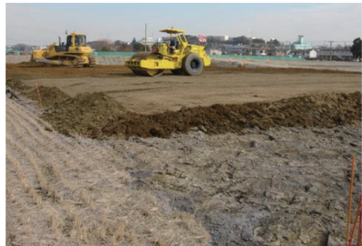
図 3.5 陸域軟弱土改良施工状況 Construction situation of the soft ground improvement
