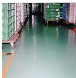
写真2 エスレベル施工後の平滑性 （エポキシ樹脂で塗装） Flatness of the floor surface using S-LEVEL (the surface is painted with epoxy resin)
