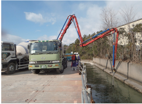
写真6 均し部の施工状況 7) View of leveling concrete by anti-washout SSHM
