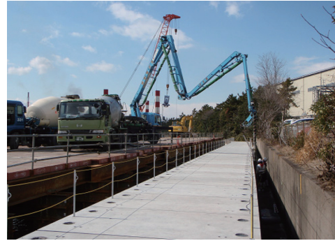
写真7 間詰め部の施工状況 7) View of filling part by anti-washout SSHM
