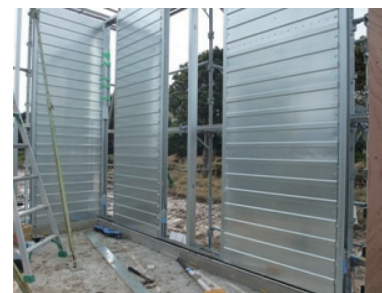
図12 折板壁 Corrugated sheet wall
