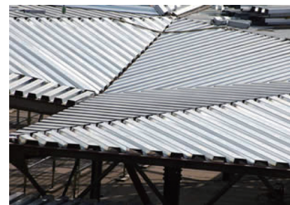
図11 折板屋根 Corrugated sheet roof
