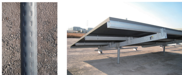
図 23 ディンプル鋼管 (左) と太陽光架台杭への適用 (右) Pipe with dimple on the surfaces (left) and an example of application for foundations of the solar systems (right)
