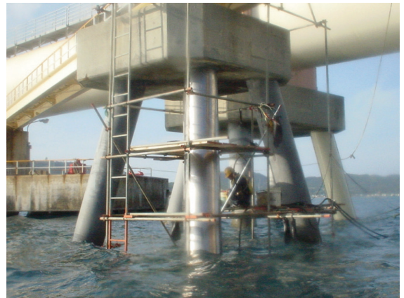
写真8 TP工法適用事例 Example of employment of TP construction method
