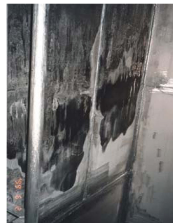
図1 粗製りん酸によるタンク内壁の黒変の一例 Example of black change of chemical tank wall by crude phosphoric acid
