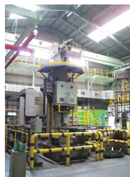
写真7 CIPの外観 Appearance of CIP
