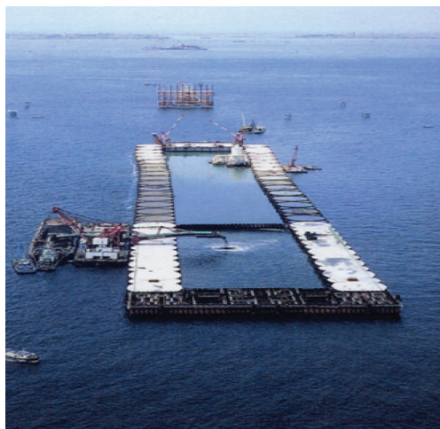
写真6 東京湾横断道路木更津人工島での周辺護岸の締め切り Revetment using straight steel sheet pile of man-made island of Tokyo Trans Bay Highway.
