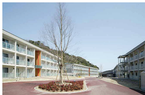
写真13 北九州市留学生宿舍(三階建・60分準耐火建築物) Three-story dormitory for foreign students in Kitakyushu city (60 minutes quasi-fire-resistant building)
