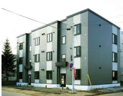
写真10 札幌市の都市型三階建共同住宅(耐火建築物) Three-story apartment, city type, in Sapporo city, Hokkaido (1 hour fire-resistant building)
