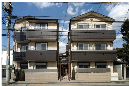
写真12 調布市の狭小地都市型三階建共同住宅(耐火建築物) Three-story apartment, city type and narrow small area, in Chofu city, Tokyo (1 hour fire-resistant building)
