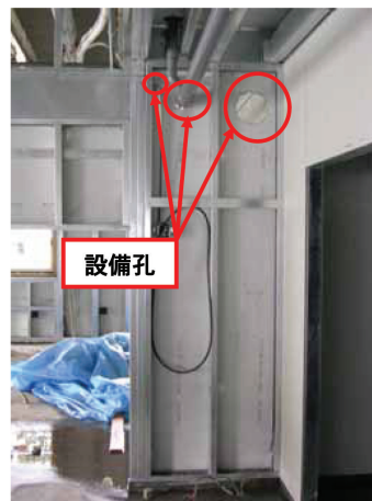
写真17 構造面材への配管貫通孔のプレノッチ化 Pre-notched holes for piping penetration to structural face board
