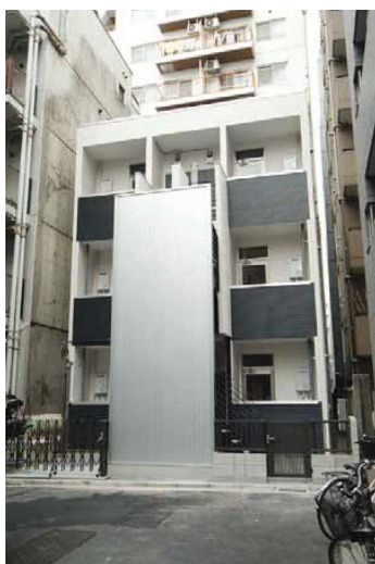
写真11 南池袋の狭小地都市型三階建共同住宅(耐火建築物) Three-story apartment, city type and narrow small area, in Minami-Ikebukuro, Tokyo (1 hour fire-resistant building)
