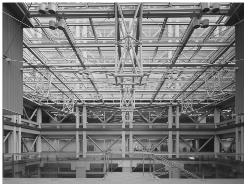
写真7 適用事例 Constructional case (atrium)
