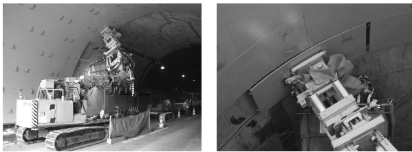
写真3 パネル設置状況 Installation of panel by elector machine
