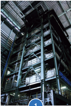
1 Annealing furnace (Vertical direct-fired reducing furnace)
