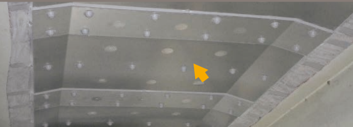
▲ Bridge reinforcing plate (steel plate adhesion method) ZAM™ ZKS processing, ZAM Grout
