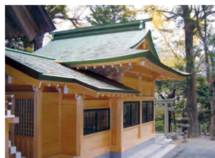
Ashitaka Shrine Surface: Alumina blasting (AD09), verdigris coloring Area: 440 m 2 Weight: 0.4 tons Completed: 2006
