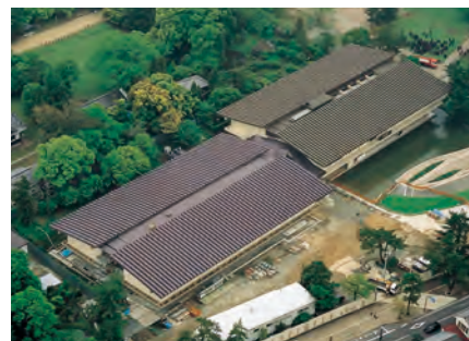
Nara National Museum (No. 2 Annex) Surface: Alumina blasting (AD03), brown coloring Area: 6,000 m 2 Weight: 12 tons Completed: 1998
