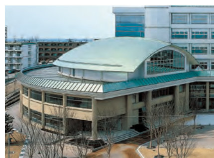
Uchinada Town Office Surface: Roll dull (ND20) (green coloring) Area: 1,700 m 2 Weight: 6 tons Completed: 1998
