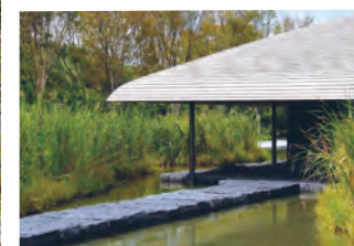
Miyajidake Shrine Surface: Roll dull (ND20) Gold coloring Area: 220 m 2 Weight: 0.86 tons Completed: 2010
