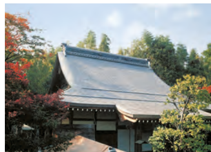
Koetsuji Temple, Main Hall Surface: Alumina blasting (AD03) Area: 700 m 2 Weight: 1.2 tons Completed: 1997
