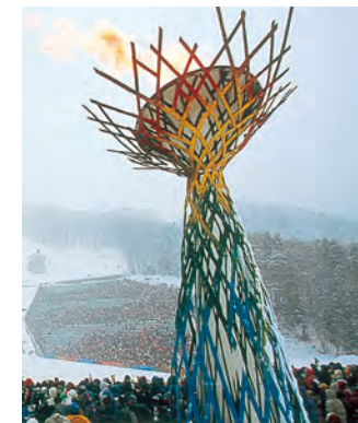
Flame Holder at the Nagano Winter Olympic Games Surface: Mirror surface Sheet thickness: 2.0, 3.0 mm Designed by: Kiyoyuki Kikutake (information sculptor) Installed by: Tig Completed: 1998
