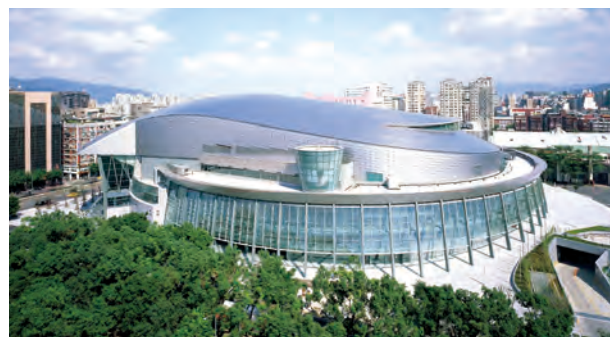
Taipei Arena (Taiwan) Surface: Roll dull (ND20) Area: 20,000 m 2 Weight: 50 tons Completed: 2007
