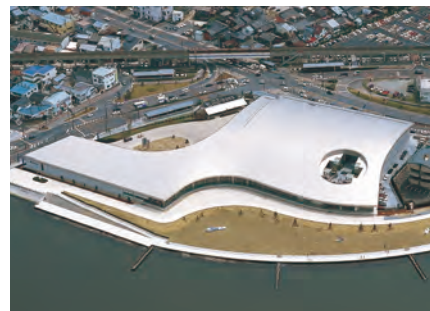
Shimane Art Museum Surface: Pickled dull (VP20), equivalent to VP15 (PD25NX (no longer offered)) Area: 10,000 m 2 Weight: 60 tons Completed: 1998
