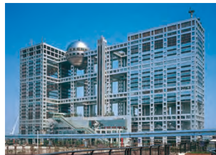
Fuji Television Headquarters, Spherical Observation Room Surface: Roll dull (ND10), equivalent to gloss SD3 (ND10 (no longer offered)) Area: 2,800 m 2 Weight: 14 tons Completed: 1996
