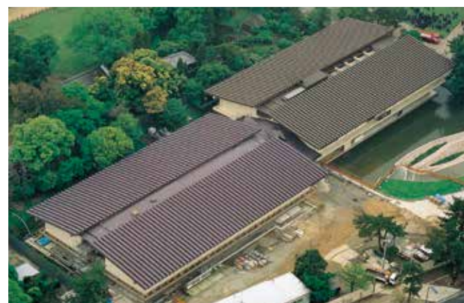
Nara National Museum (No. 2 Annex) Surface: Alumina blasting (AD03), brown coloring Area: 6,000 m 2 Weight: 12 tons Completed: 1998
