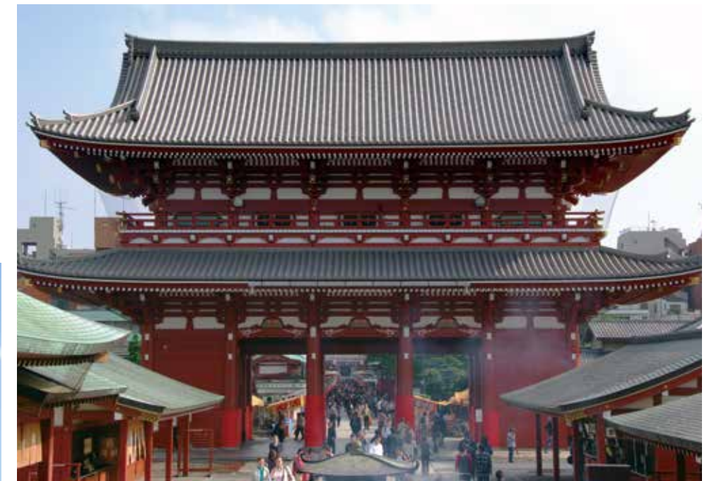
Hozomon of Sensoji Temple Surface: Alumina blasting (AD03, AD06) Area: 1,000 m 2 Weight: 8 tons Completed: 2007
