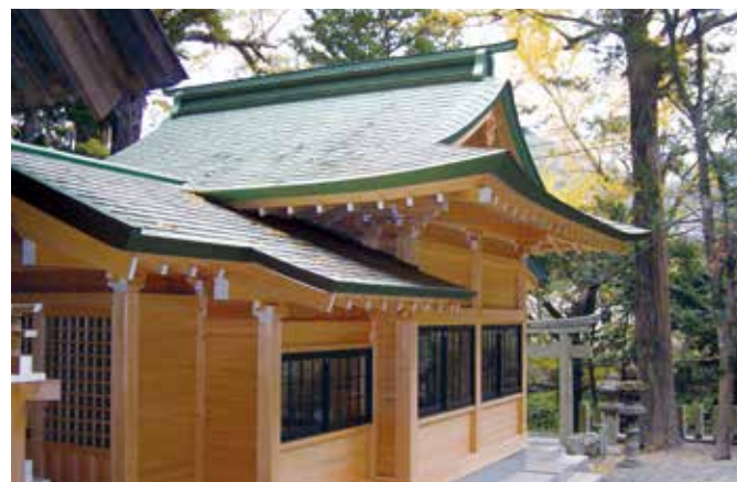
Ashitaka Shrine Surface: Alumina blasting (AD09), verdigris coloring Area: 440 m 2 Weight: 0.4 tons Completed: 2006
