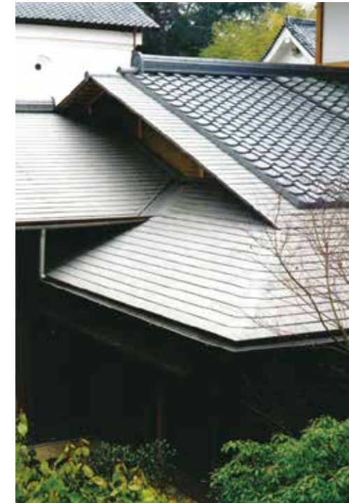
Teahouse (Josokutei) of Kinkakuji Temple Surface: Alumina blasting (AD03) Area: 100 m 2 Weight: 0.5 tons Completed: 2003
