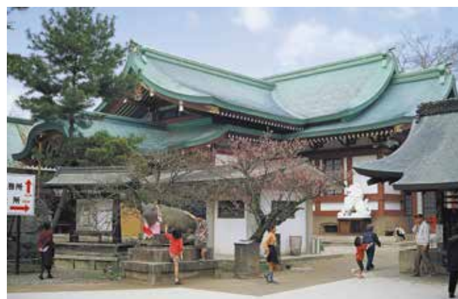
Kitano Tenmangu/Treasury Surface: Alumina blasting (AD09), verdigris coloring Area: 1,000 m 2 Weight: 4 tons Completed: 1998
