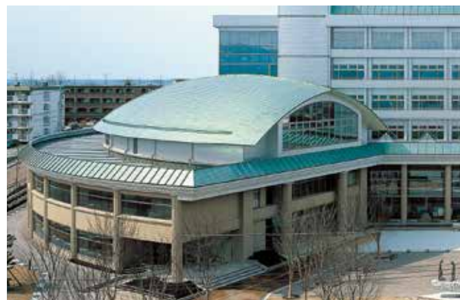
Uchinada Town Office Surface: Roll dull (ND20), green coloring Area: 1,700 m 2 Weight: 6 tons Completed: 1998
