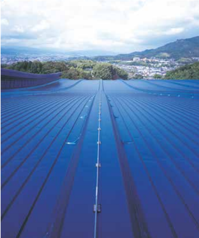
Application of edge waves ⇒ Rolling (with ribs) ⇒ Seam welding
