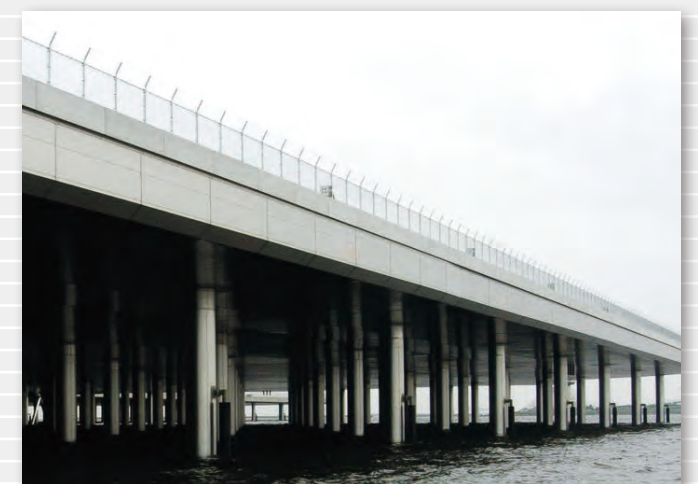
Tokyo International Airport D-runway pier
