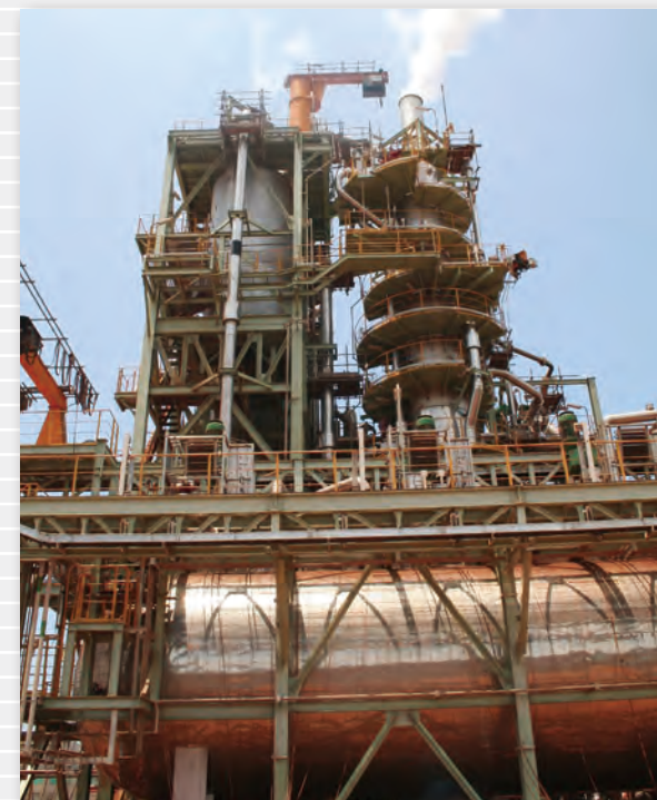
General view of wet-type Nickel Refining Plant
