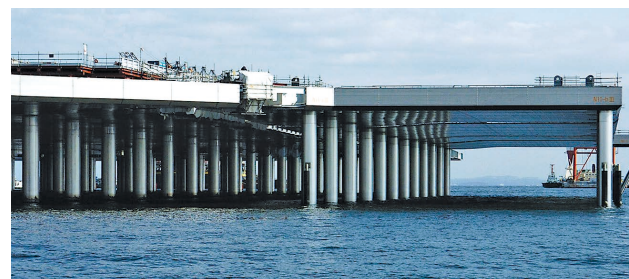
Pipe piles for large offshore platforms
