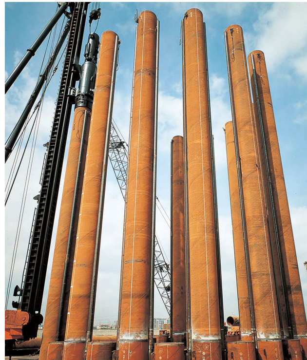
Pipe sheet piles for earth-retaining structures
