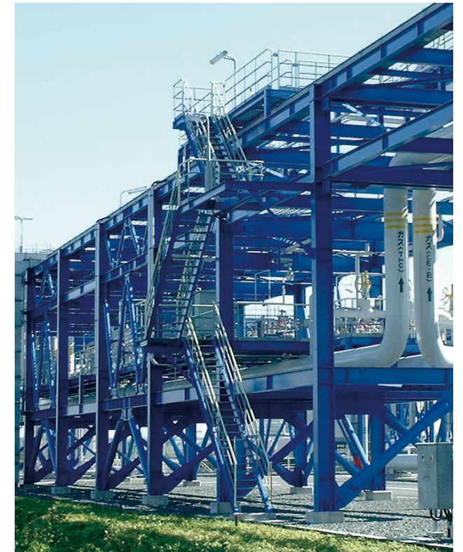
In-plant gas piping
