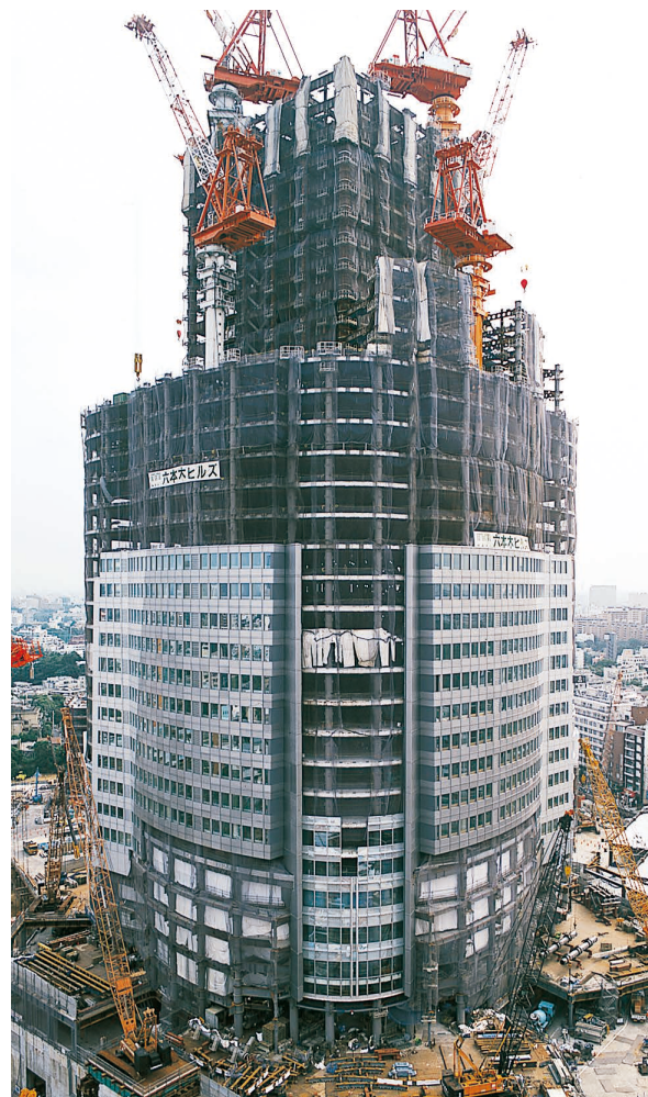
Pipe & tube columns for high-rise buildings
