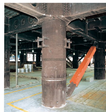
Pipe & tube columns for high-rise buildings
