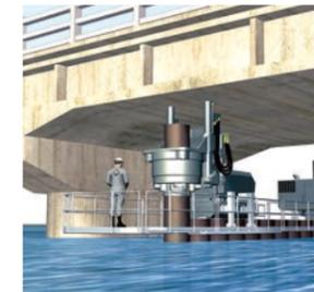
Easy installation at a place with limitation in overhead clearance.
