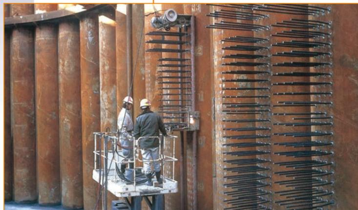
Example of the shape of a steel pipe sheet pile joint (P-P joint: 165.2 mm (φ) × 11 mm (t))
