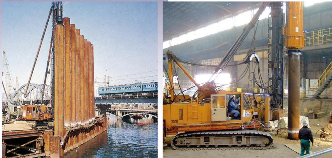
A construction method in which vibratory hammers are used to forcibly apply vibration to piles to temporarily reduce pile shaft friction and edge indentation resistance during installation.
