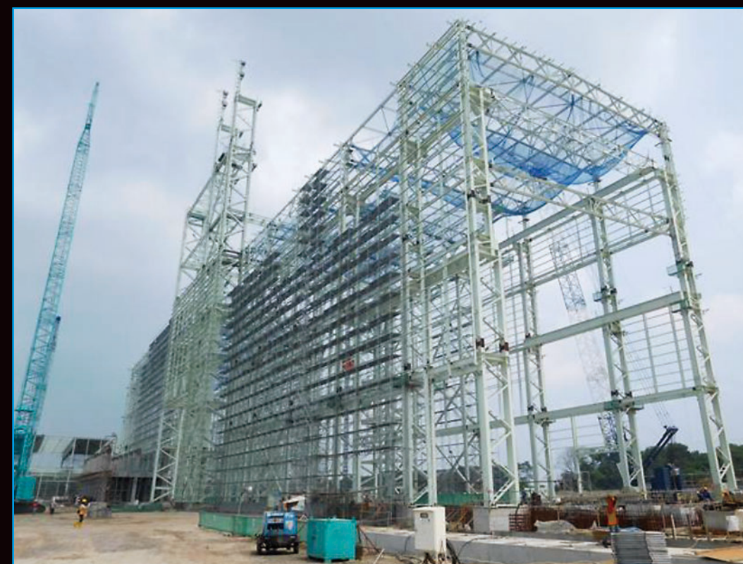
[Steel Finishing Plant] Country : Indonesia Product : NSHYPER BEAM™
