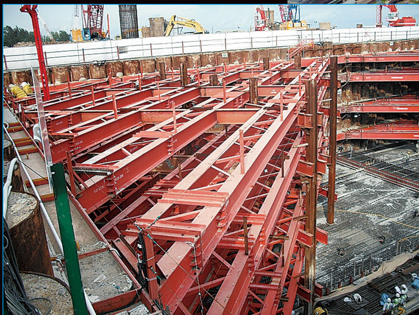
[Temporary Retaining Wall] Country : Singapore Product : NSHYPER BEAM™ UC356x406 series
