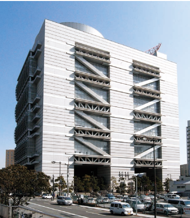
Conference center (application of steel Unbonded Braces)
