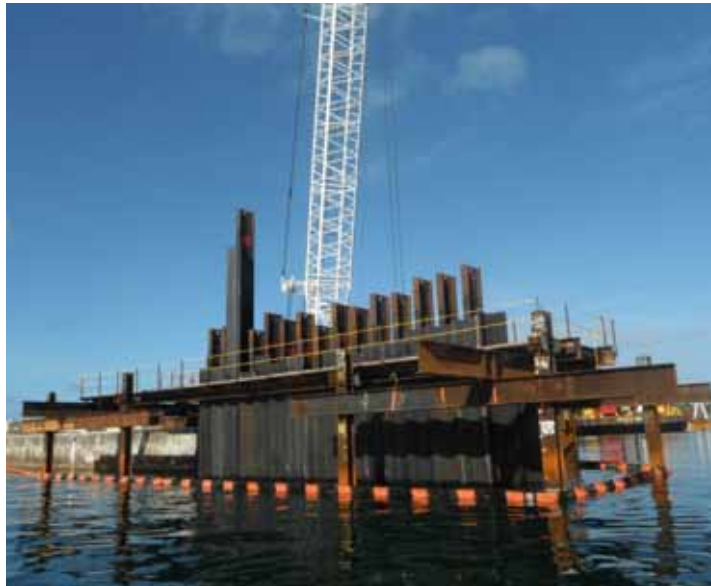
(1) “Hat + H” shown during the process of construction
