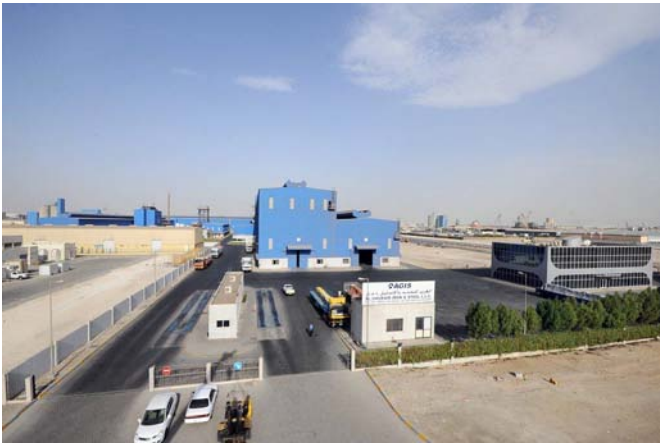
▲ Entrance of AGIS plant
