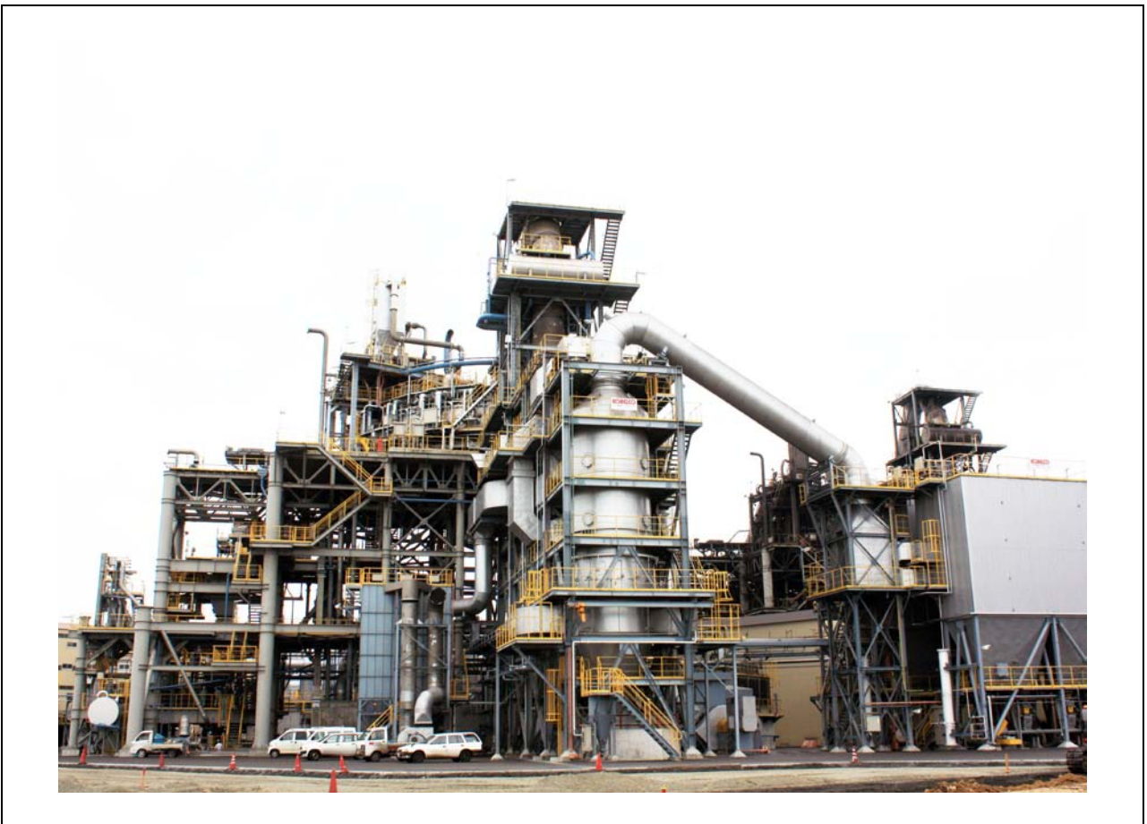
Nittetsu Shinko Metal Refine's steel dust recycling plant
