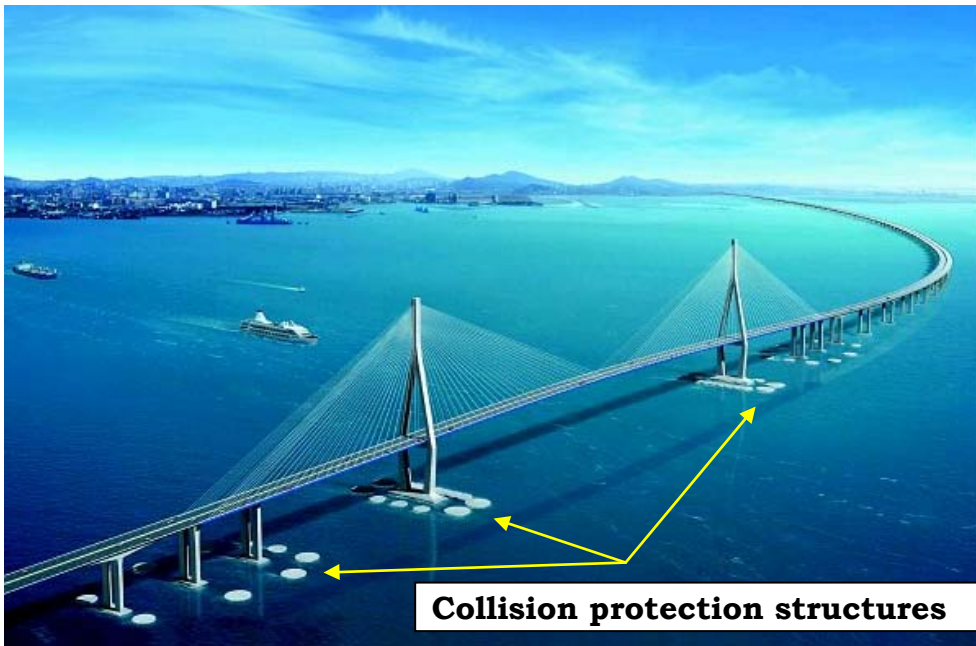
Fig. 1: Artist's sketch of the collision protection structures in service (Courtesy: Construction department of Samsung C & T Corp.)
