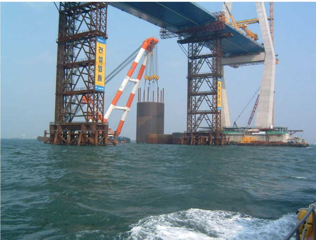
Fig. 4: Photo showing the cell under construction (Photographed by Nippon Steel)
