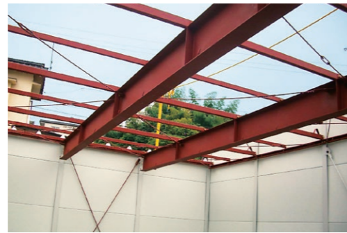
Adoption of SMart BEAM™ for constructing a convenience store
