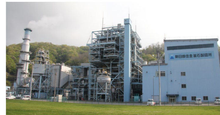
Kamaishi Works coal-fired thermal power plant
