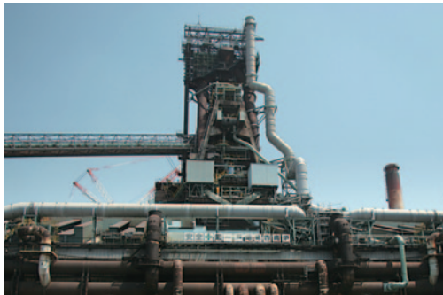
Reinforcing domestic manufacturing bases
