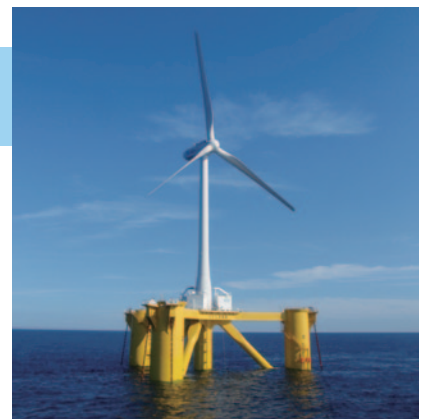
2 MW downwind-type floating offshore generation facility "Fukushima Mirai" (approx. 80 meters in windmill diameter) © Fukushima Offshore Wind Consortium
