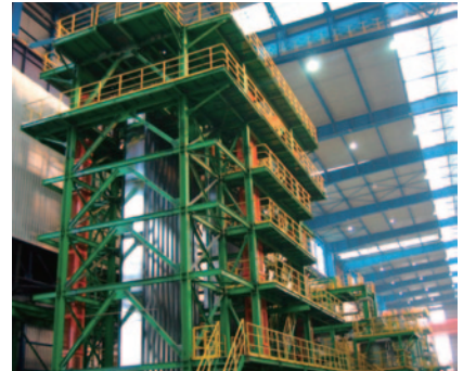
WINSteel's electrolytic tinning facility
