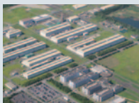
Research & Engineering Center (Futtsu)
