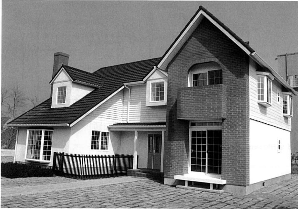
Photo 3 Application on test steel house (Kashima Messe)
