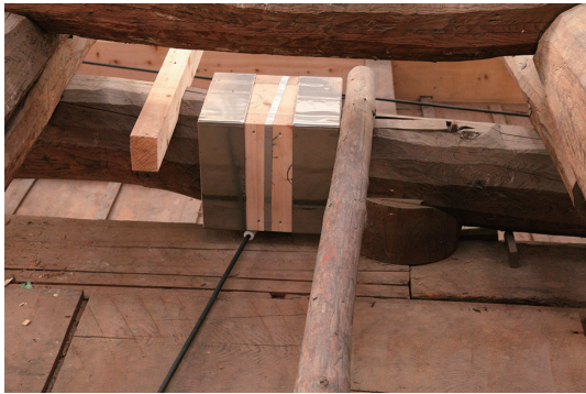
Photo 2 Titanium alloy sheet wrapped member shown in Photo 1
