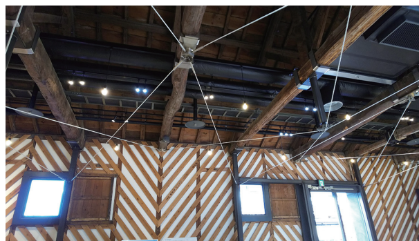
Photo 7 Reinforcement of Tomioka Warehouse No.3
