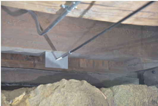
Photo 4 Reinforced member joint of structure shown in Photo 3 (using titanium alloy bolt)
