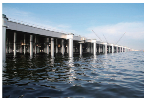
Fig. 1 Application of stainless steel sheathing to offshore steel structures
