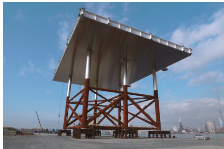
Fig. 13 Jacket structure
