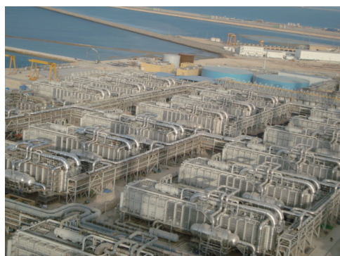
(b) Seawater desalination plant (S31803, S32304)
