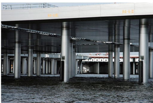
(a) Haneda Airport stainless steel lining jacket (NSSC 270)
