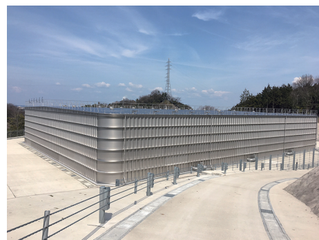
(b) Water supply tank in Yonago (SUS329J4L, SUS316, SUS304)
