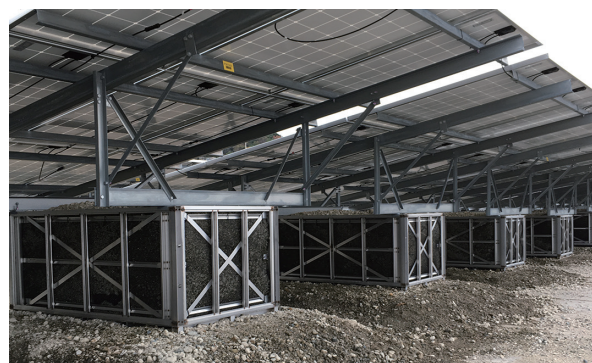
Photo 6 Application of FW to solar panel mount
