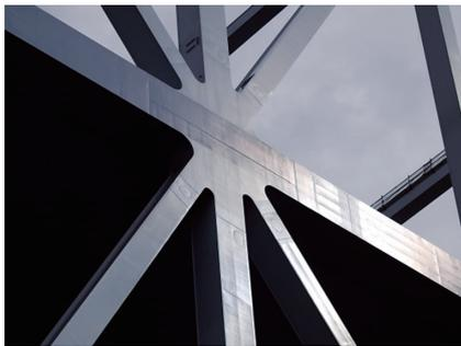
Photo 4 Example of the panel points on the Tokyo Gate Bridge
