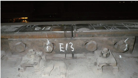
Photo 6 Insertion of a cut rail
