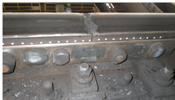
Photo 5 Damaged rail joint
