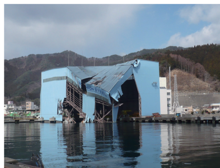
Photo 5 Partially destroyed all-weather berth
