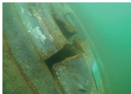
Photo 3 Damage to second tie-rod
