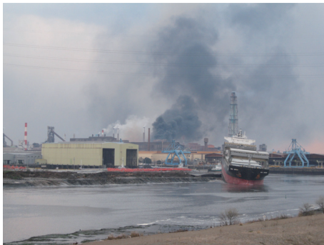
Photo 11 Damage to shore protection facilities due to collision with a vessel by the tsunami
