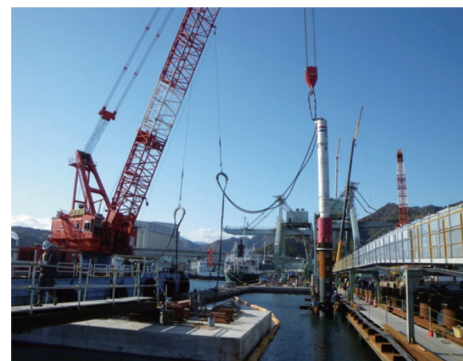
Photo 6 Piling by flying hammer method
