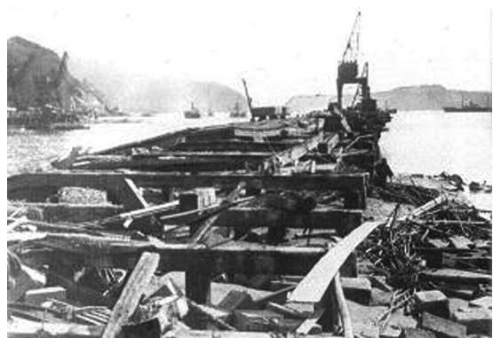
Photo 4 Pier completely destroyed by a tsunami
