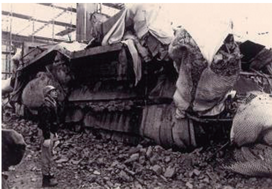
Photo 13 Reinforced concrete structure after blasting demolition
