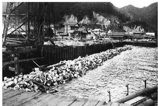
Photo 3 Use of steel sheet piles for shore protection (circa 1937 in Kamaishi)
