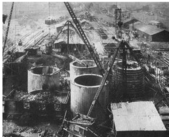
Photo 5 Sunk-well foundation for blast furnace in Kukioka
