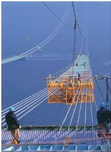
Photo 12 Cable installation for Akashi-Kaikyo Bridge
