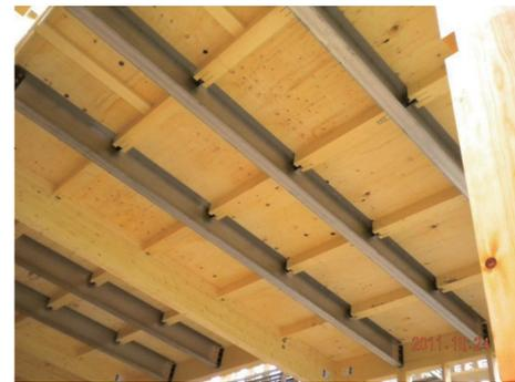
Fig. 7 Application case of “SMart BEAM” construction method
